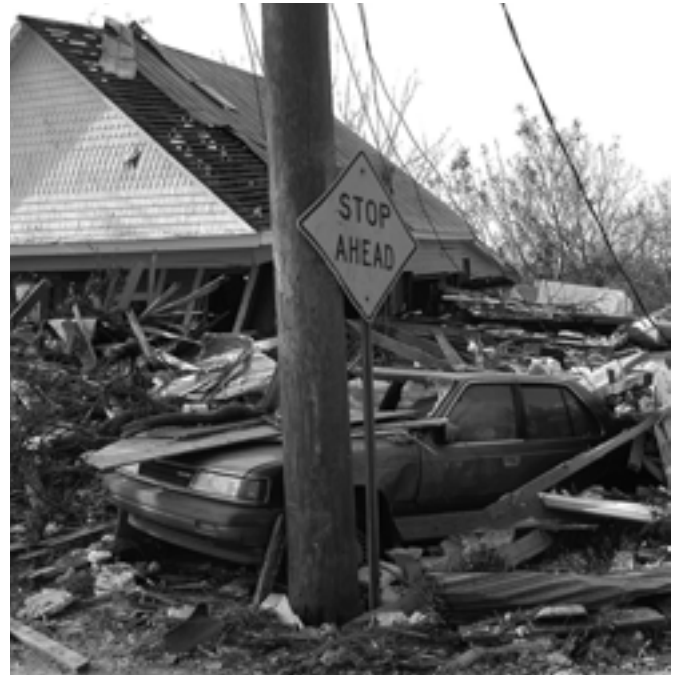
Katrina aftermath: houses transformed to debris, Gulf Port, MS. Photo: Christopher Kyle Craig.
