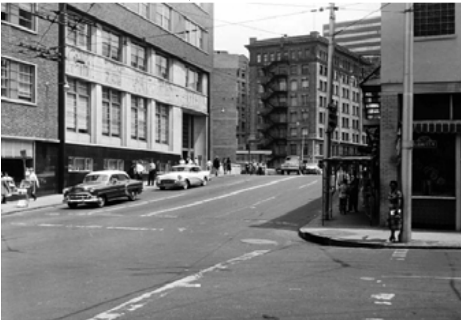
View of Constitution Building entrance and Julian Harris mural at Forsyth Street, Special Collections Department, Pullen Library, Georgia State University.
